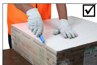
Step 1: Cut the polythene film
