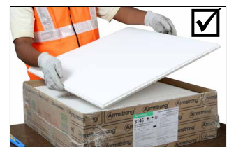
Step 3: Remove the tile
